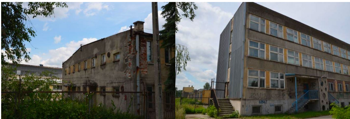
Figure 78. Former Plastics Processing Plant, Kłaj / Source: GPR for the district of Kłaj for 2017-2025
