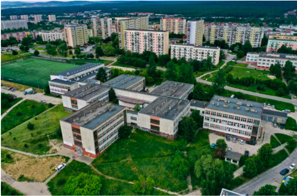
Figure 20. Top view of the former school complex on Jana Nowaka-Jeziorańskiego street in Kielce / Source: Municipal Building Management in Kielce.
