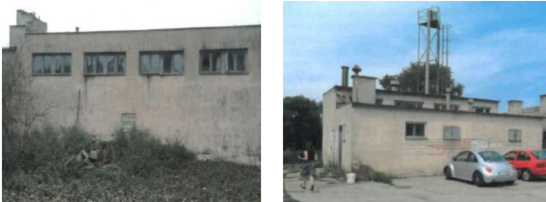
Figure 36. former steam boiler plants in the Tuchola district / Source: Local Revitalization Program for the Tuchola District for 2016-2023, pp. 29-32.
