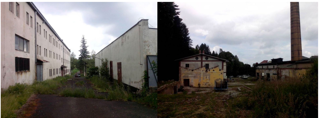
Figure 30. Post-factory buildings in the town of Lešna, Pobiednia / Source: Local Revitalization Program of the Lešna Commune for 2016-2023, p. 59.
