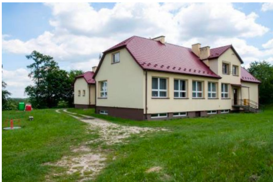
Figure 53. Building of the former school in Dąbrówka, Pleśna district /Source: GPR for the Pleśna district for 2016-2023
