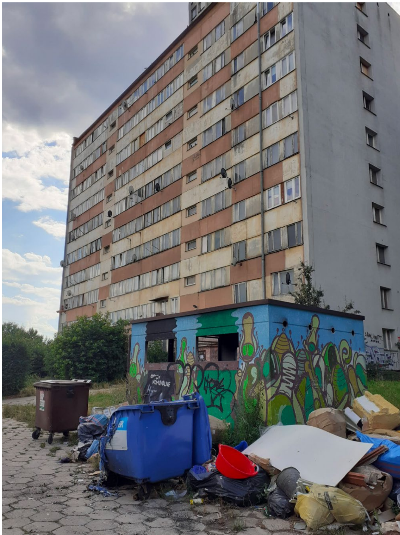
Figure 17. The building at Mtodej Street in Kielce / Source: IRMiR
