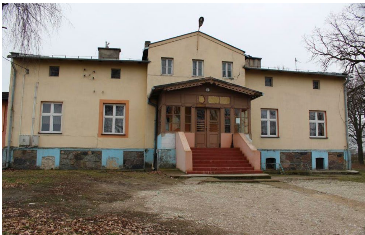
Figure 39. Former school building, Szczkowo, Izbica Kujawska / Source: Local Revitalization Program for the district of Izbica Kujawska for 2017-2023, p. 63 (photo: E. Sulczyńska).
